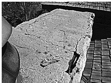
Damaged Chimney Cap
