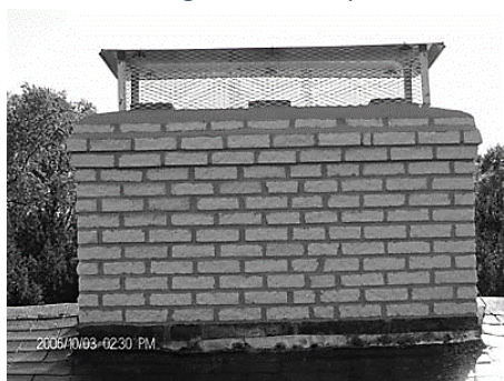
Metal Cap on Clay Liner Chimney Top
