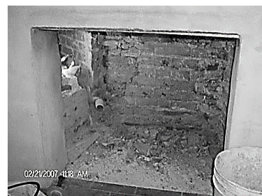
Badly Deteriorated Firebox
