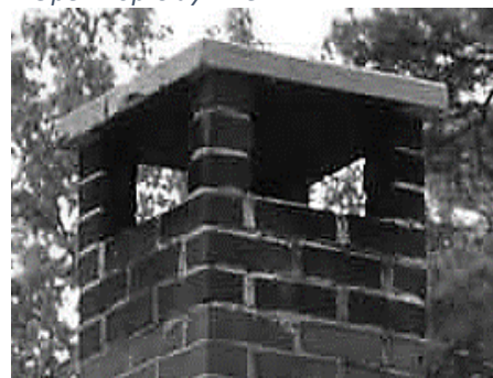
Concrete Cap Chimney Top
