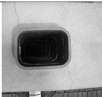
Clay Tile Liner Flue
